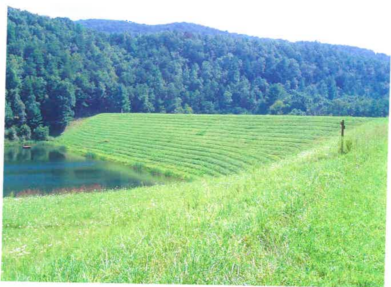
Todd Lake Dam (UNR 10) – Augusta County, VA
